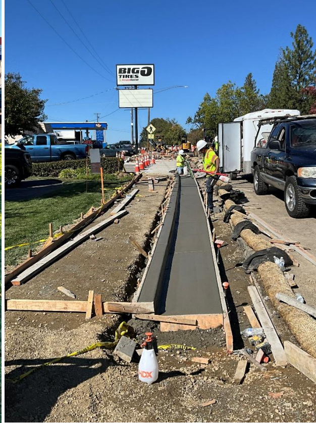
Pouring Curb and Gutter
